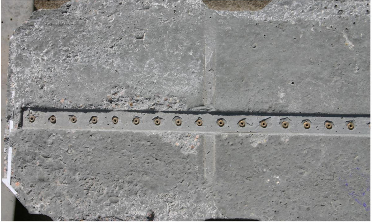
Figure 4.2: Embedded brass points used for Whittemore readings
