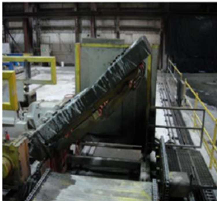
Figure 3.9: Vacuum lifting of ties
