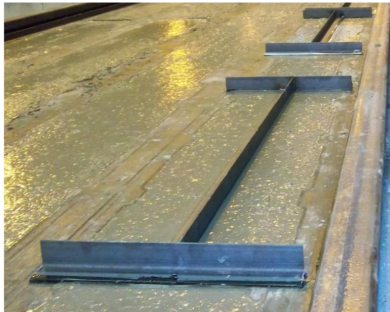
Figure 3.13: Steel bars cast in fresh concrete
